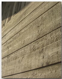
BOARD FORMED CONCRETE
