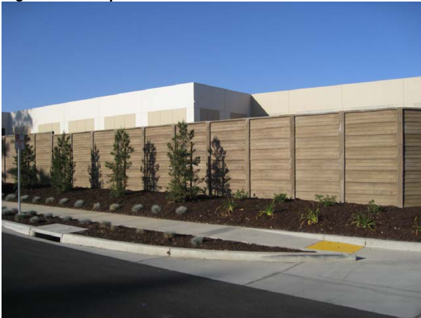
Figure 4: Example of sound wall
