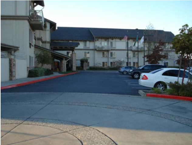
Figure 1: Photo of area proposed for pool addition and related improvements.
