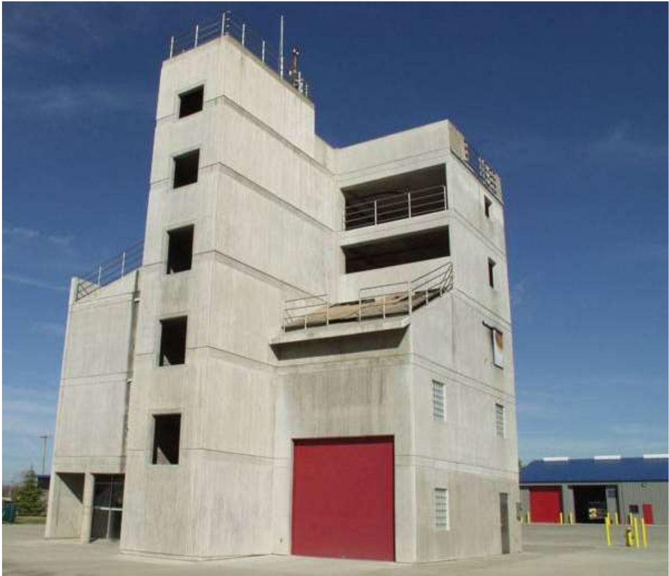
Figure 13-5. City of Roseville Fire Training Center
