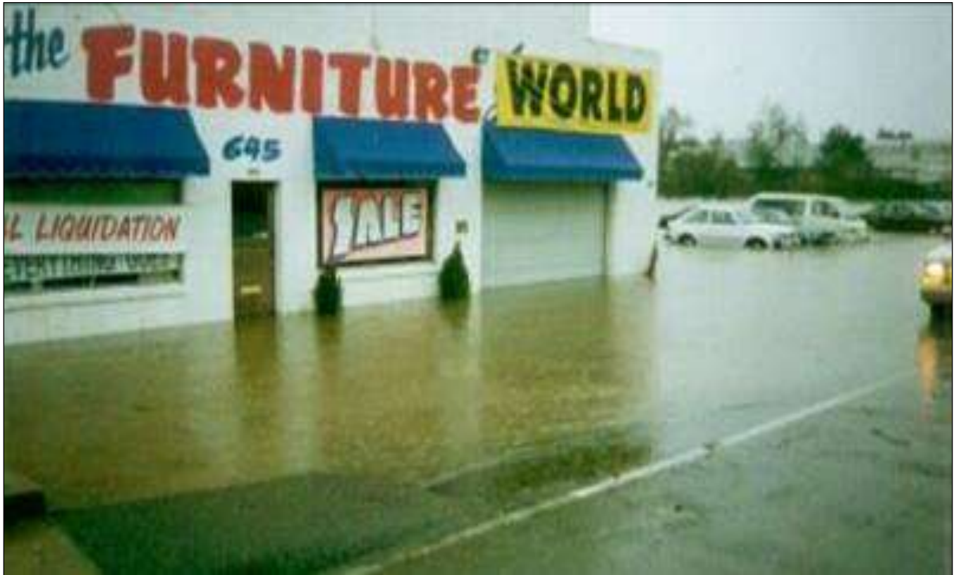
Figure 10-3. Business Flooding, February 1998
