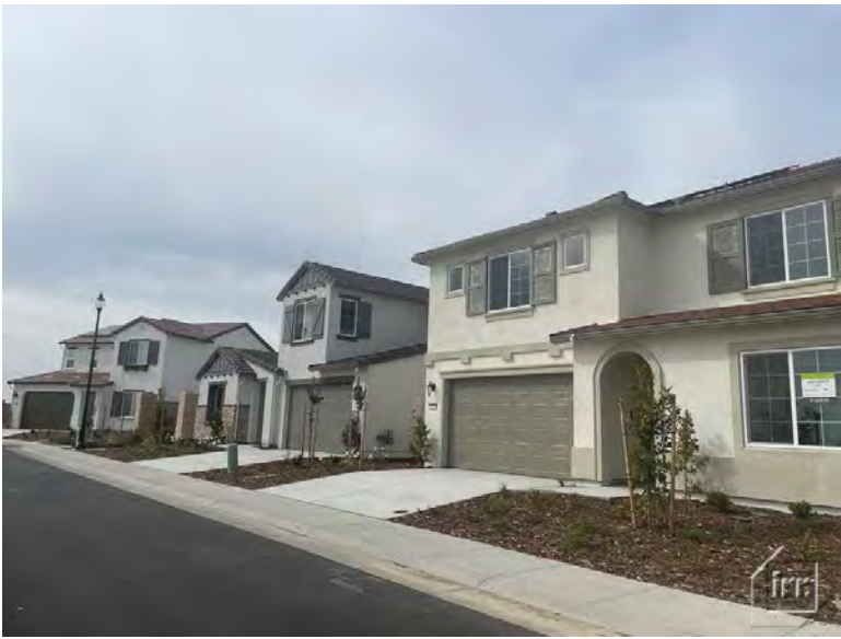
City of Roseville Westbrook CFD No. 1 Pleasant Grove Blvd. Roseville, California
