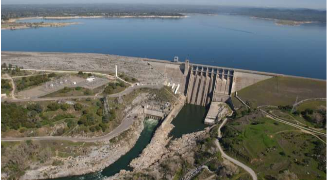
Figure 7-1. Folsom Dam and Folsom Lake on the American River, Looking Northeast
