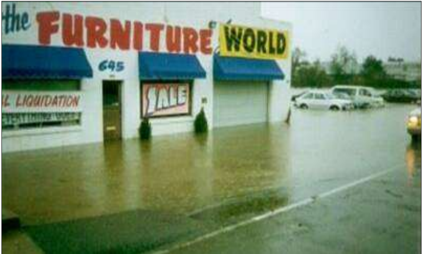
Figure 10-3. Business Flooding, February 1998
