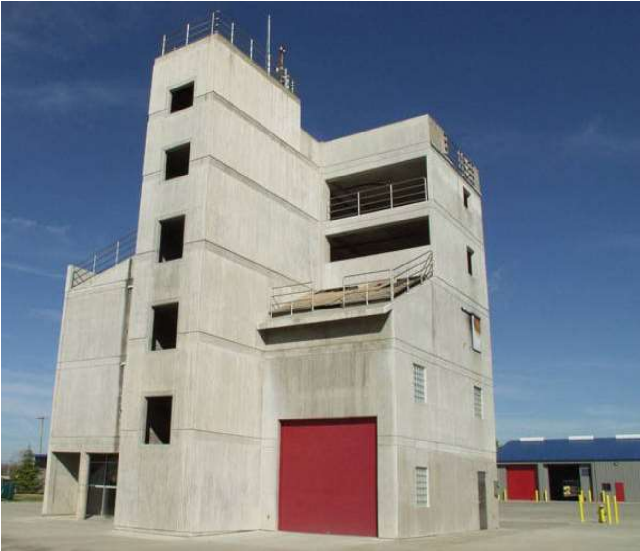
Figure 13-5. City of Roseville Fire Training Center
