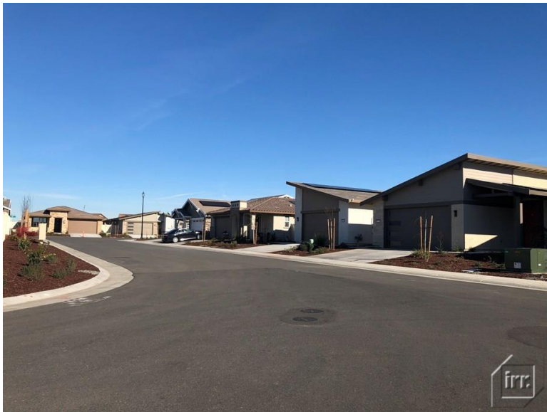
City of Roseville Westbrook CFD No. 1 South and North of Pleasant Grove Blvd Roseville, California
