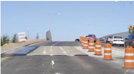
side view of the decking
