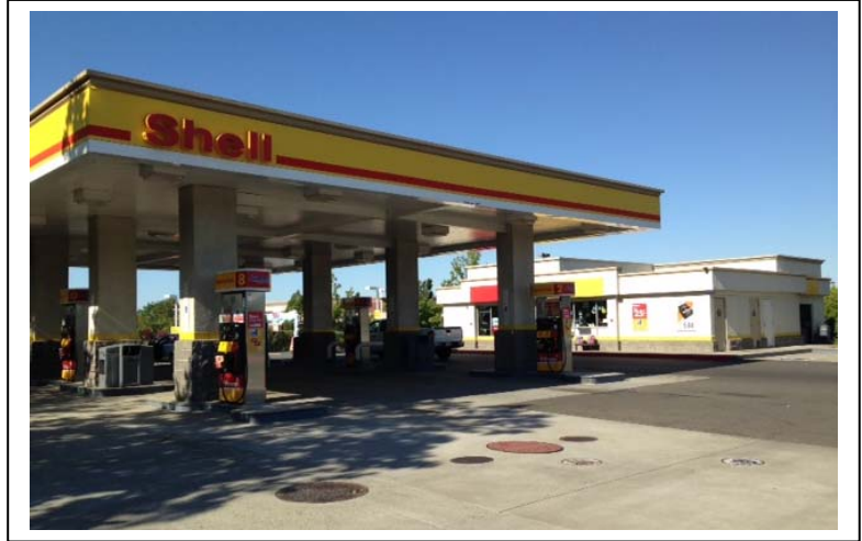
Figure 2 – Existing Shell Station
